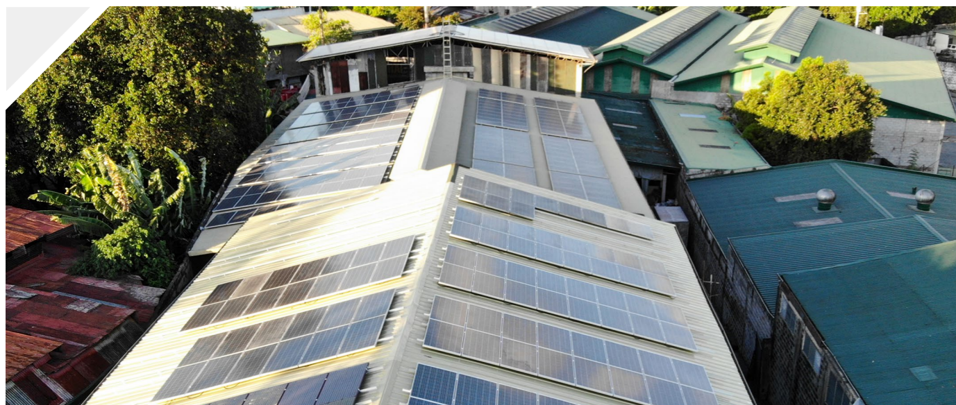
Project Address: Silang Cavite, Philippines Project Capacity: 64.8kW Inverter: 2 sets of Sunways STT 33kW inverter
