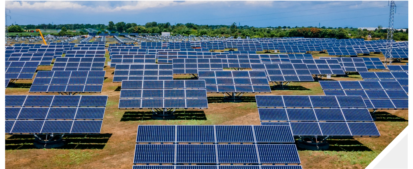
Project Address: Udine, Italy Project Capacity: 6.6MW Inverter: 522 sets of Sunways STT 12kW inverter
