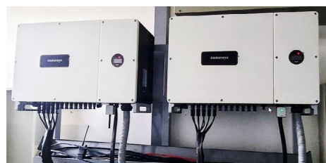
Project Address: Silang Cavite, Philippines Project Capacity: 64.8kW Inverter: 2 sets of Sunways STT 33kW inverter
