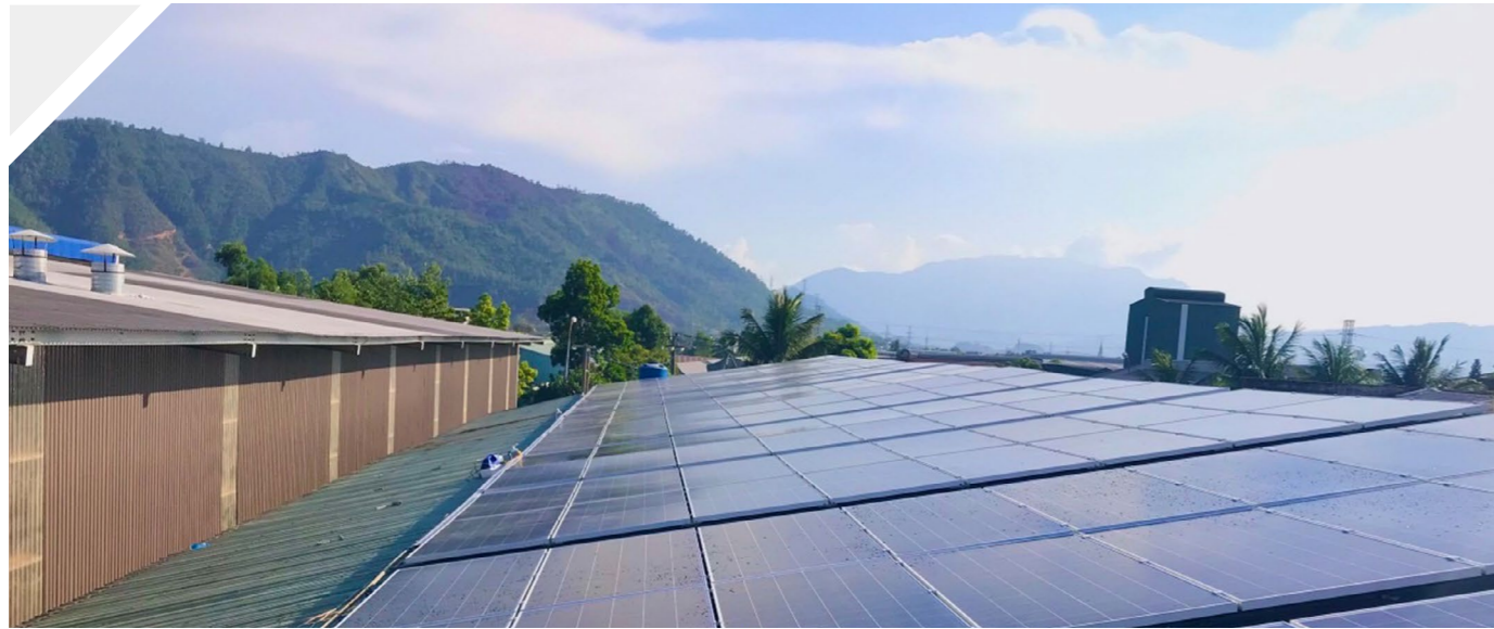
Project Address: Danang, Vietnam Project Capacity: 100kW Inverter: 4 sets of Sunways STT 25kW inverter
