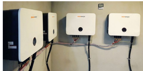
Project Address: Danang, Vietnam Project Capacity: 100kW Inverter: 4 sets of Sunways STT 25kW inverter
